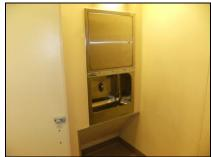
As a result, the sensor basins were incorporated in the new building designs and installed in the suburbs of Royal Oak, Manukau, Botany Downs and Lynfield. The first installations of these basins were made from resin based Aakronite. After six years in operation, it was found that these Aakronite basins were being damaged by the cleaning regime which called for basins to be scoured with an abrasive pad regularly.
