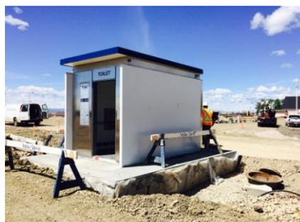
As the temperature in Calgary can get as low as  $-40^{\circ}\text{C}$ , all of the toilet units built for this environment incorporate additional insulation to all of the walls and ceilings, underfloor heating, trace wire lagging to the water supply system and large ceiling fan heaters in the main cubicle and service area to ensure safe operation of the toilet units throughout the year.
